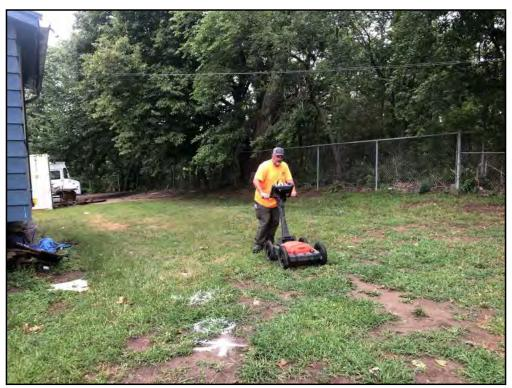
3 : Northwest- View of GPR survey near the reported former heating oil tank location (SB-3/TMW-3).
