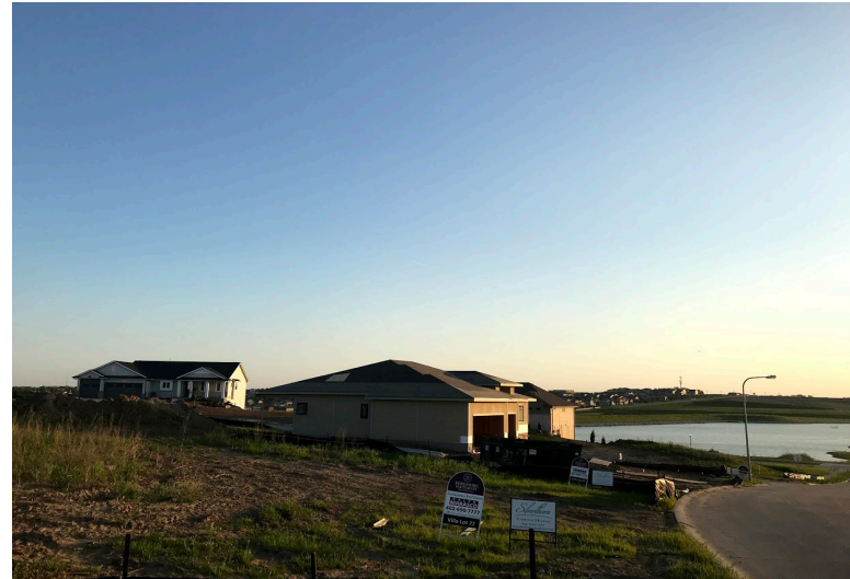
Pier 15 N 168 St & Fort St
